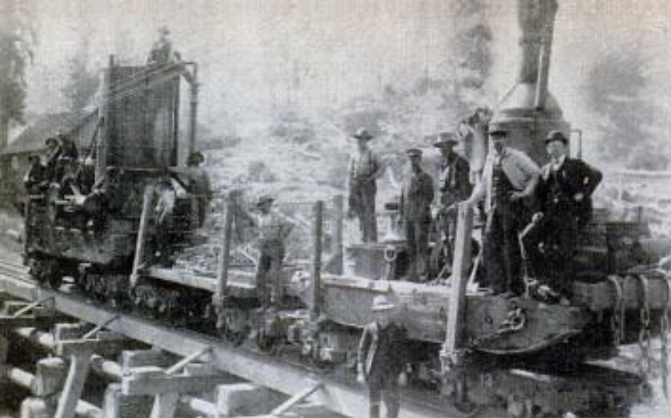
This was a big moment—the arrival of two new “donkeys.” Their cables were snagged around stumps and the donkeys pulled themselves off cars
